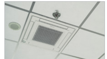
Integrates easily into the 600 x 600 ceiling tile, enabling lights, speakers and sprinklers to be installed in adjoining tiles
