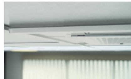
Can be installed fully flat into the ceiling, leaving only 8mm visible
