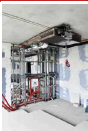
Guestroom installation (low noise slim ducted unit FXDQ)
