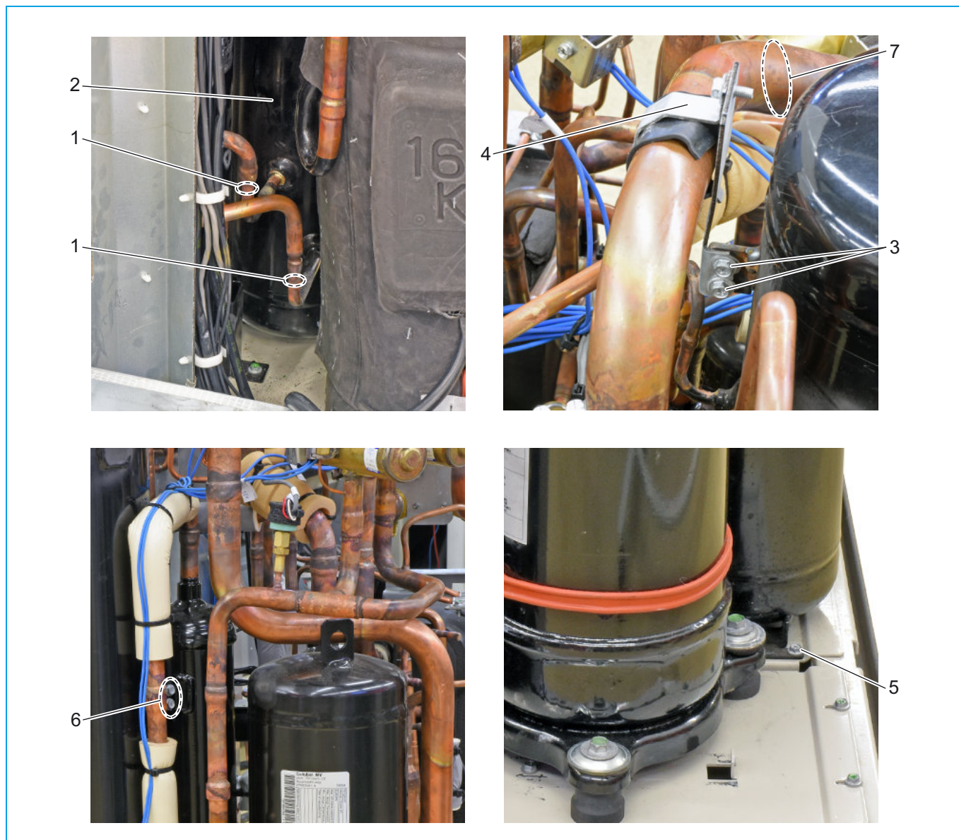
Figure 3-23: Removing the liquid receiver
