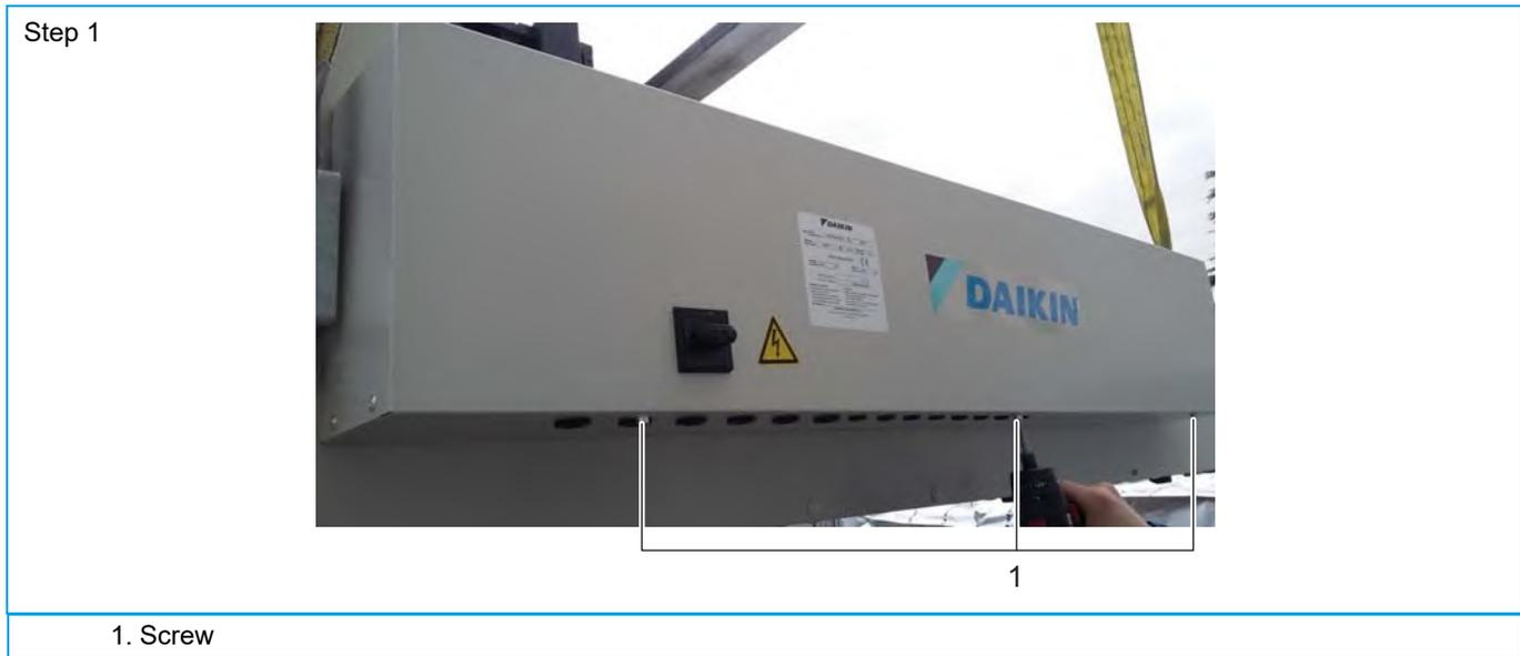
Figure 3-2: Pulling the switchbox cover
