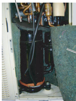
Remove the COMPRESSOR COVER A and TOP.
