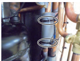
Thermistor (Discharge)
