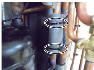
Thermistor (Discharge)
