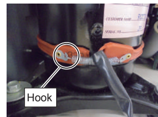
HEATER (CRANK CASE)
