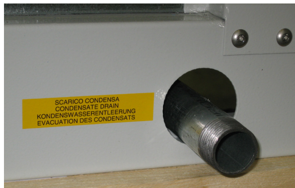
Fig. 7 Connection to the condensate collection tray
